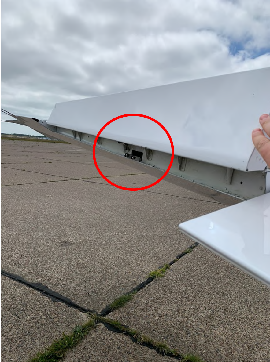
Fig. 1: Missing link to the aileron trim tab
