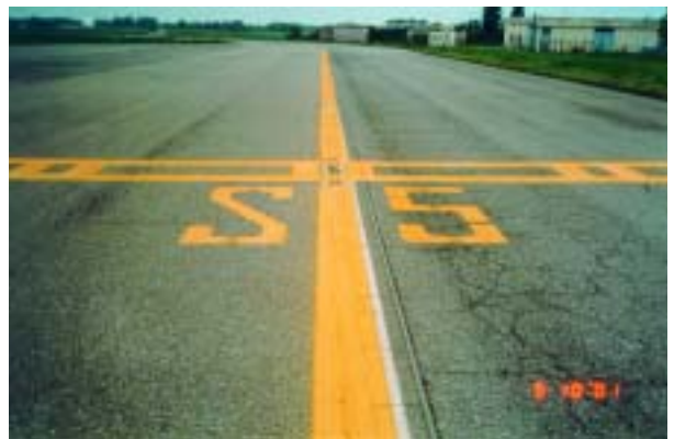
Photograph 10 - S5 marking and ICAO pattern B runway - holding.
